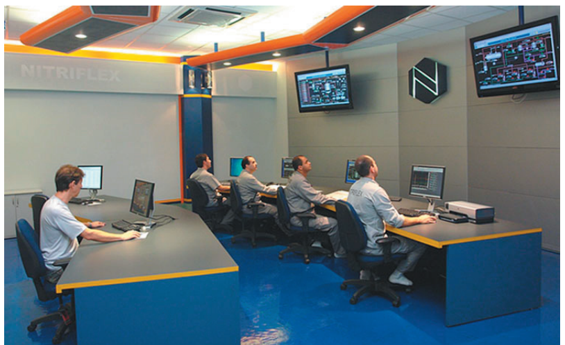
The central control room today
