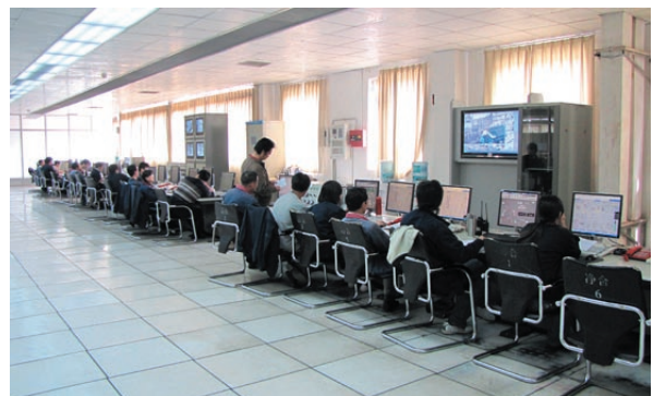
Central control room
